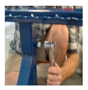
Once you have all the sections connected, insert the bolts into the nuts and tighten with a wrench.
